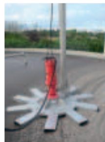
Installation of a submersible aerator type SCLK.
