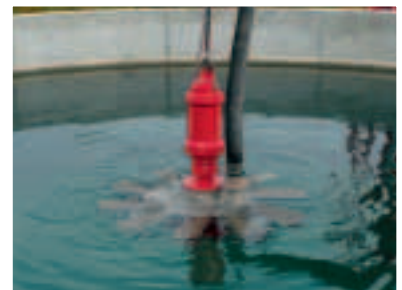
Immersion stages of a submersible aerator type SCLK.
