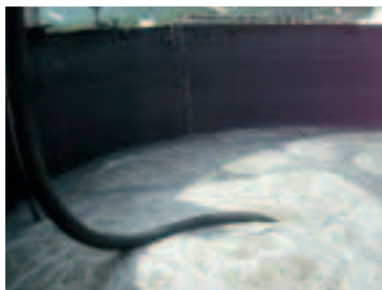
Submersible aerator type SCLK working inside an oxidation tank.
