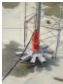
Installation of a submersible aerator type SCLK.
