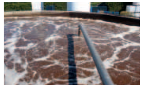
Submersible aerator type SCLK working inside an oxidation tank.
