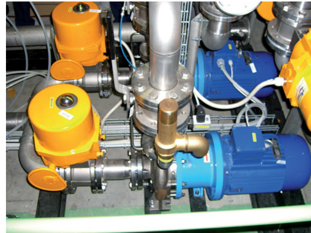
The mag drive pumps have an extended choice of materials as well as a wide variety in models. With its 100% zero leakage mag drive coupling the mag drives are your problem solvers in fluids and chemicals transfer.
